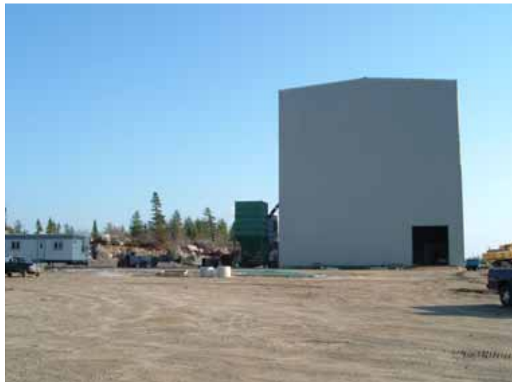
Completed Processing Building
