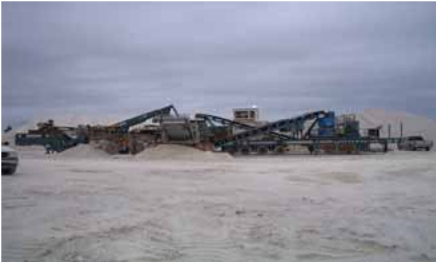
Crushing Pit-Run Material to Feedstock
