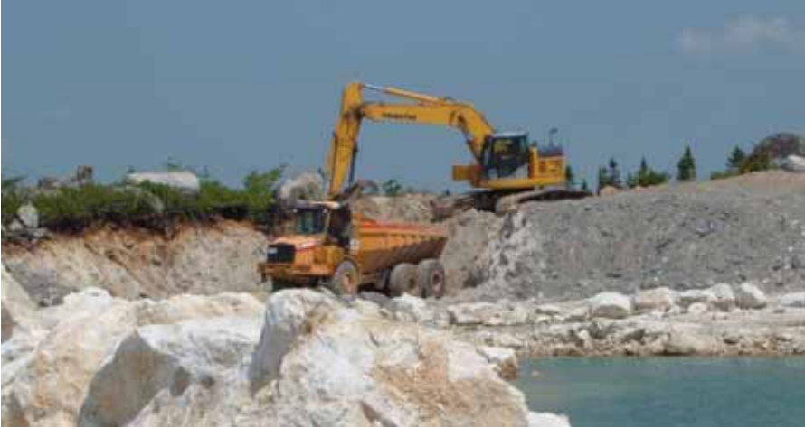
Preparation for Blast and Crush Commenced with Overburden Removal
