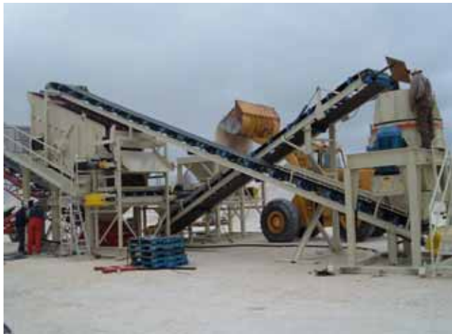
Barmac VSI Crushing System in Full Operation
