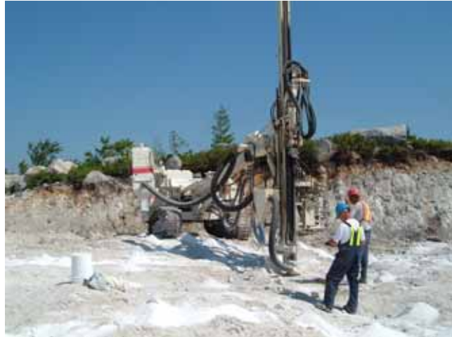
Drilling in Preparation of the Blast
