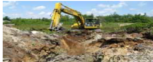
Kaolin Sample Excavation
