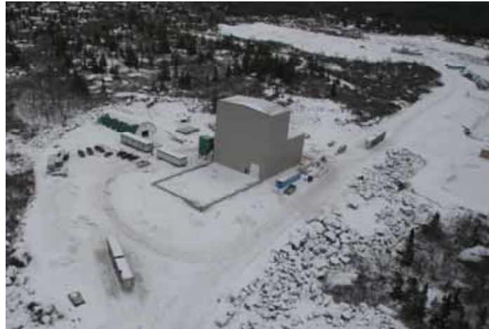
Plant Expansion in Progress (December 7, 2007)
