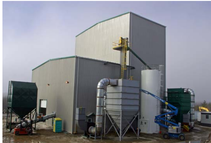
Plant Equipment Installation & Commissioning (Photo by Linda Ross)
