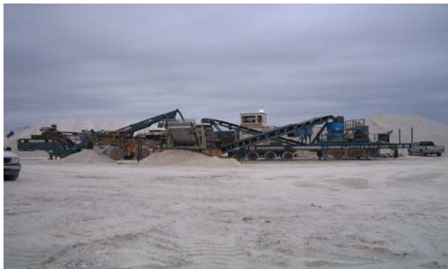
Crushing Pit-Run Material to Feedstock
