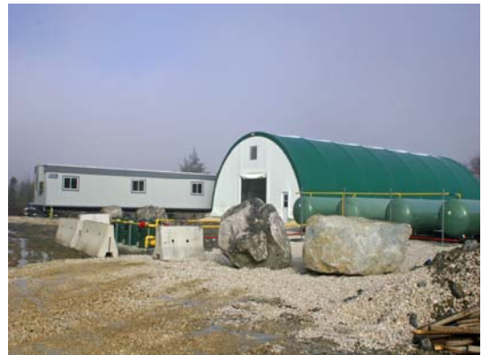
Office Trailer, Storage Building, & Fuel Storage (Photo by Linda Ross)
