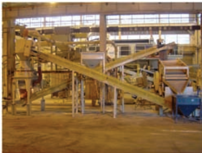
Barmac Crushing Plant
